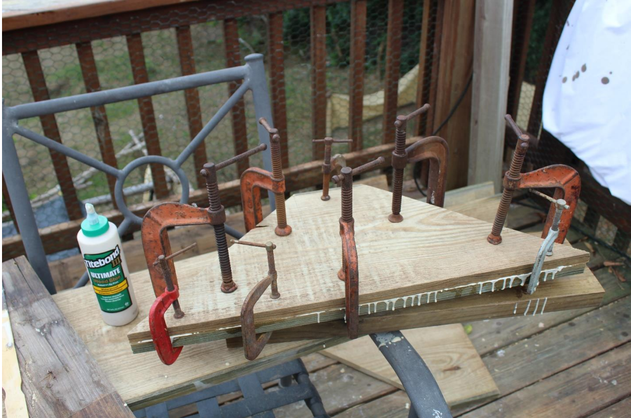
Laminating the cantilever supports for the arch-shelf and the bench
